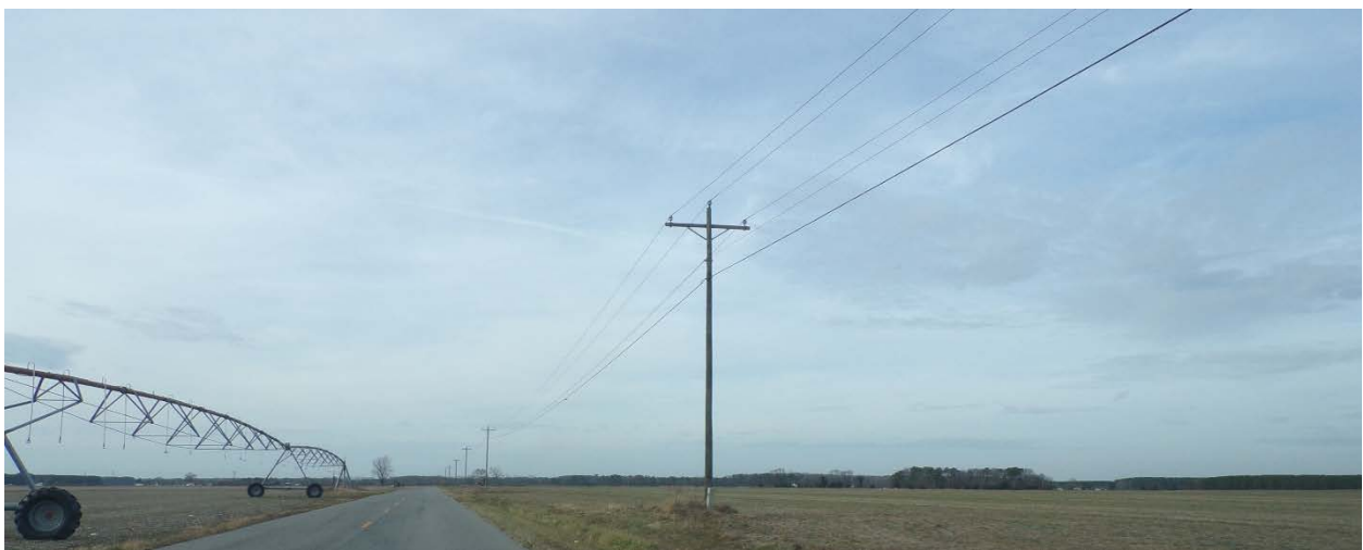
Figure 18: Low-Make-Ready Pole Line in Unserved Area
