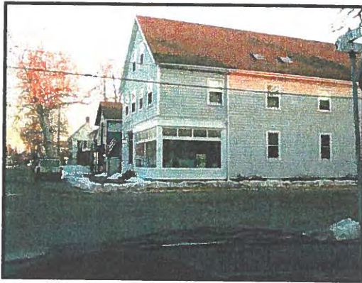
Adaptive reuse suits in-town commercial development
