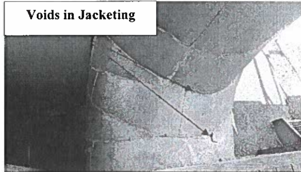
Photograph #5 – Exterior Metallic Ductwork
