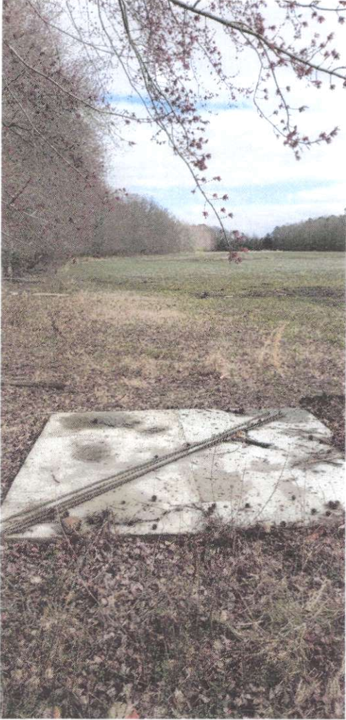
Shows concrete pad that will be used for unloading food waste before being mixed with carbon and organized into piles. Piles will be in uniform sections on opposite side of pad. (see exhibit 4 for layout of piles)
