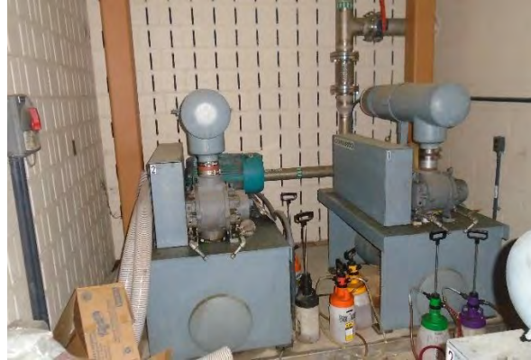
Photo 3: Process Blowers Needing Variable Speed Drives
