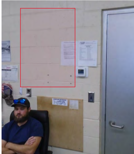
Photo 6: Location for New MBR Control Panel
