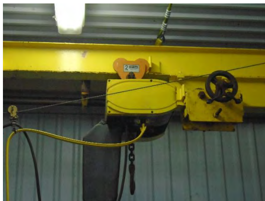
Photo 1: Hoist And Crane Over Membrane Tank
