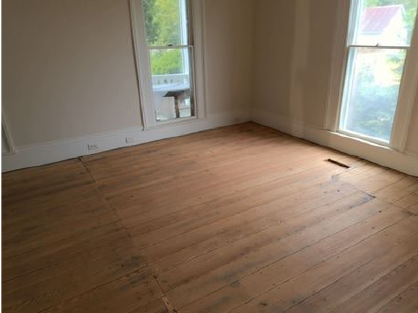
Additional dining room area - #4
