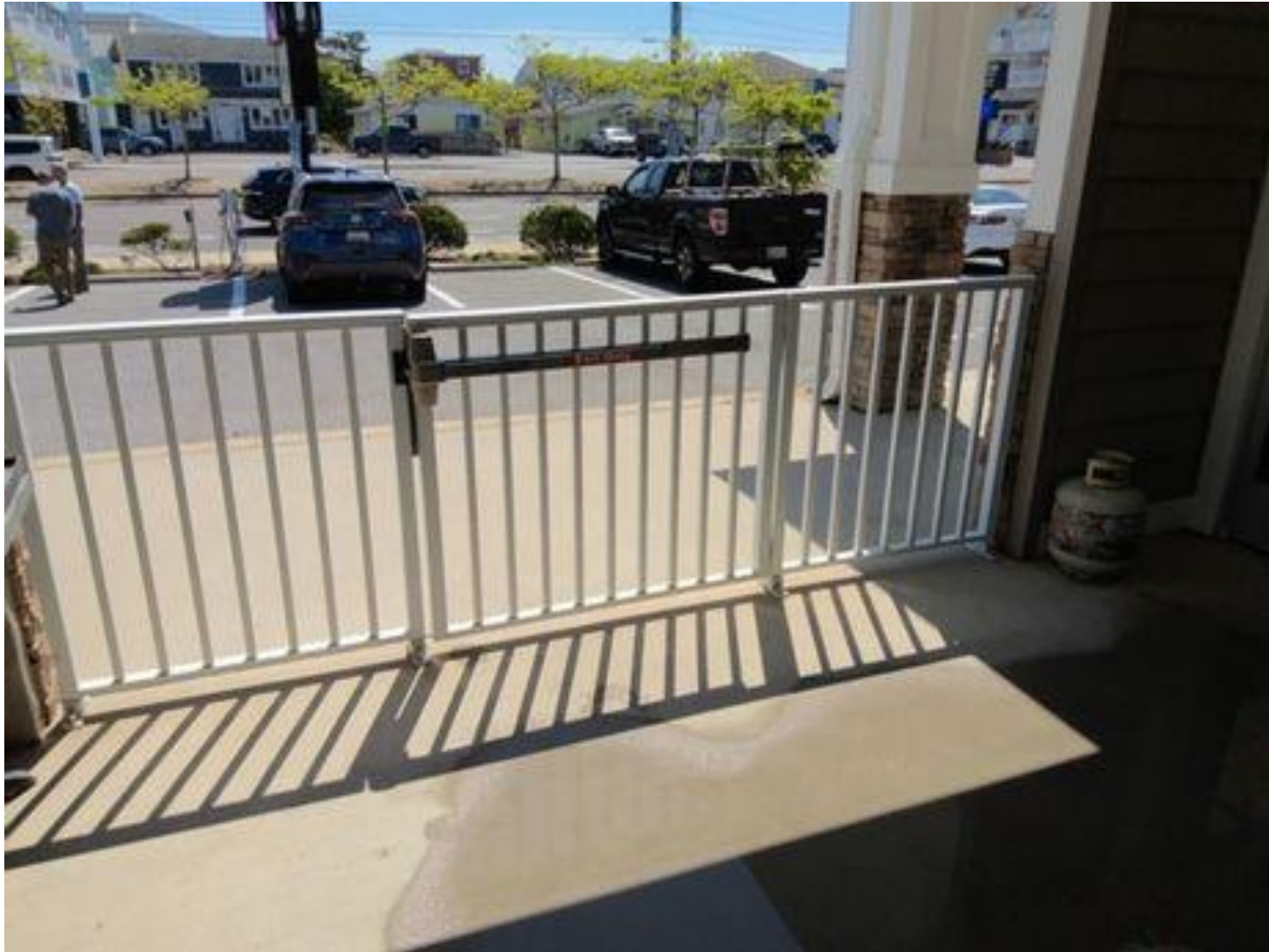
Picture of gate going to parking lot on the first floor
