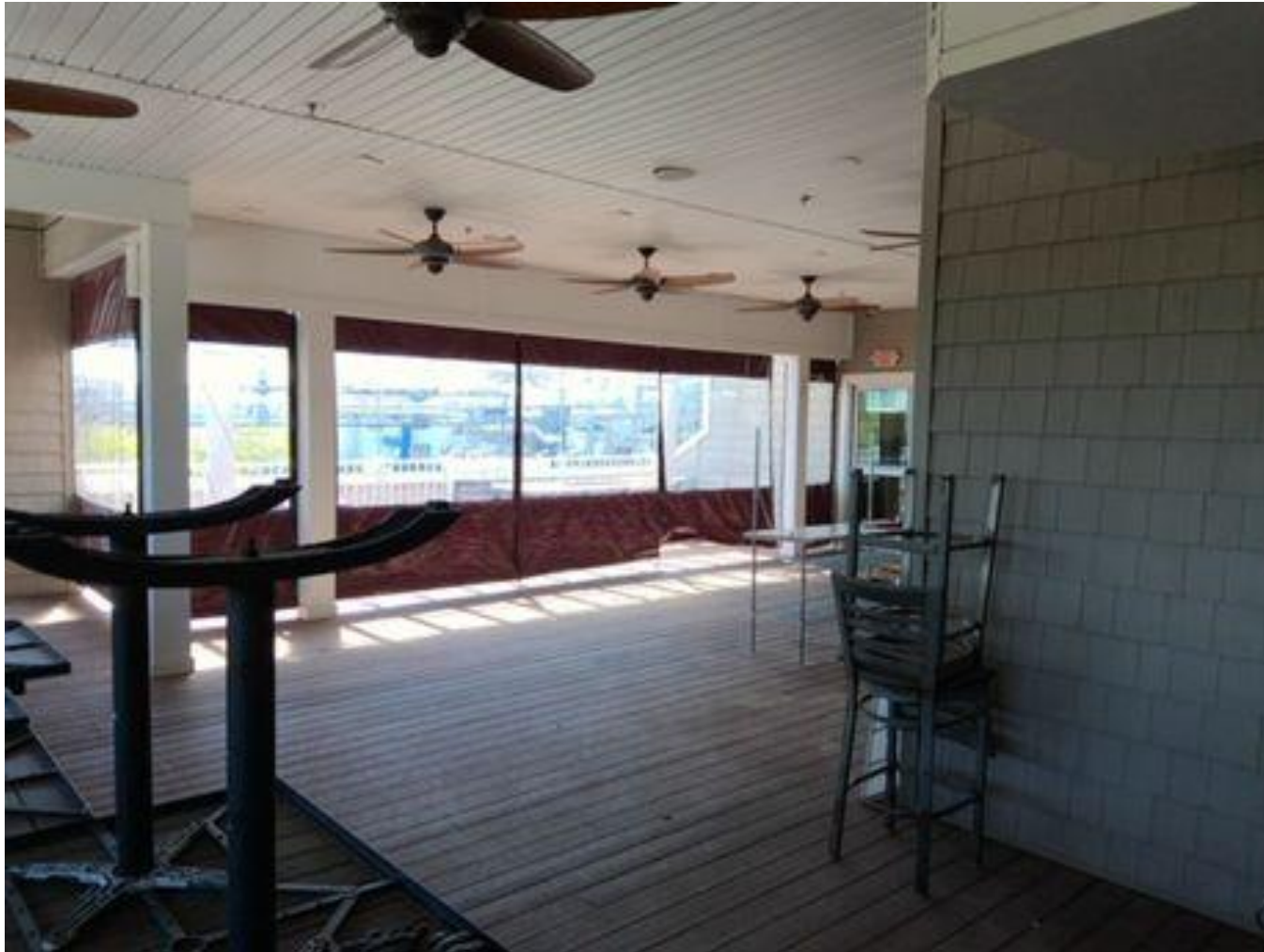
Second floor area looking from top of steps
