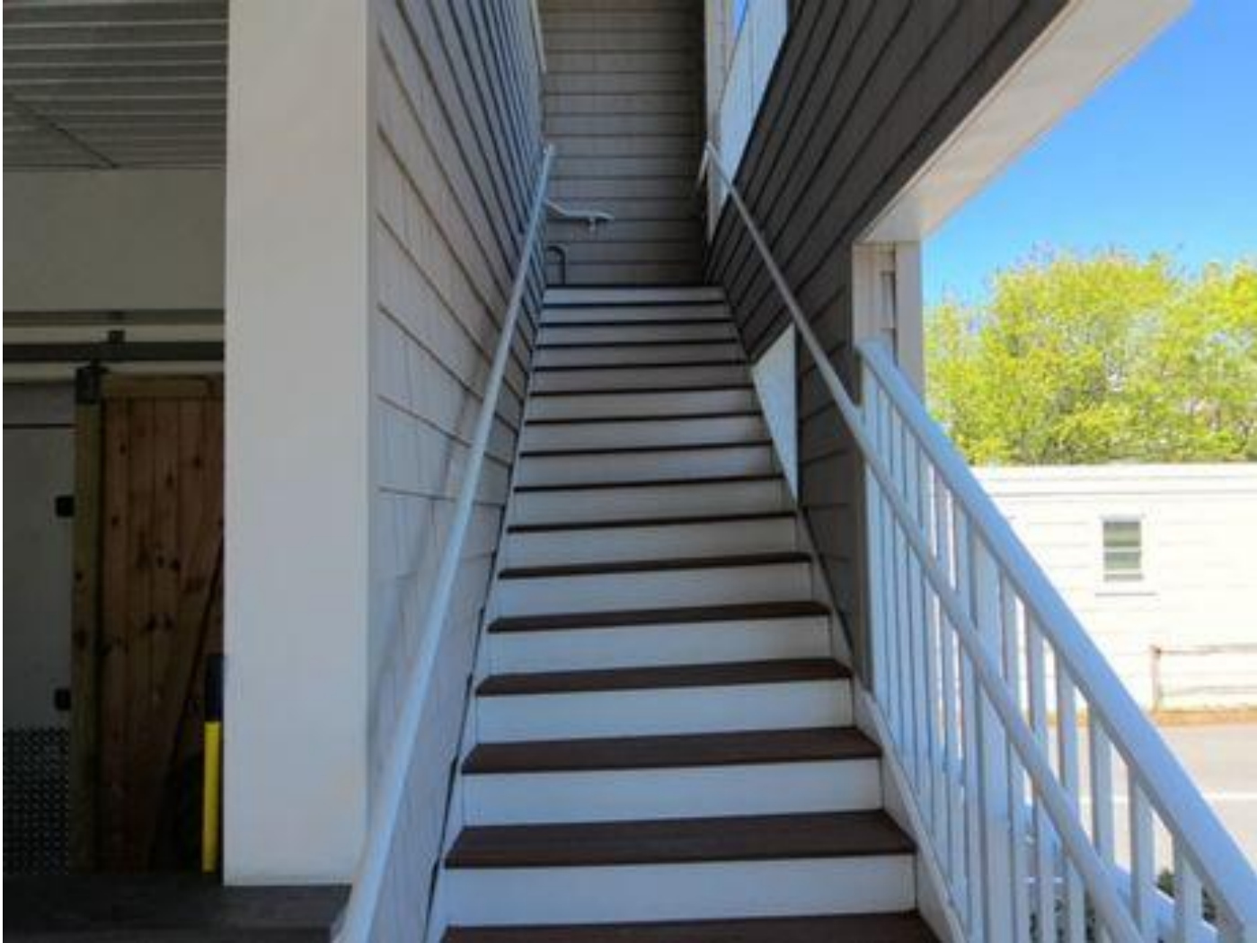
Exterior steps going from first floor to second floor
