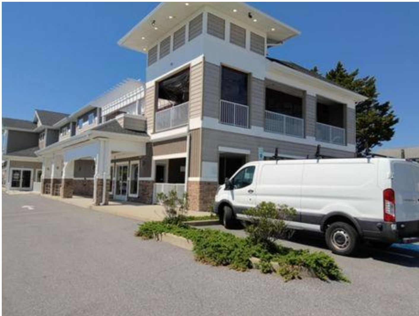
Looking to the front entrance from 79 TH Street
