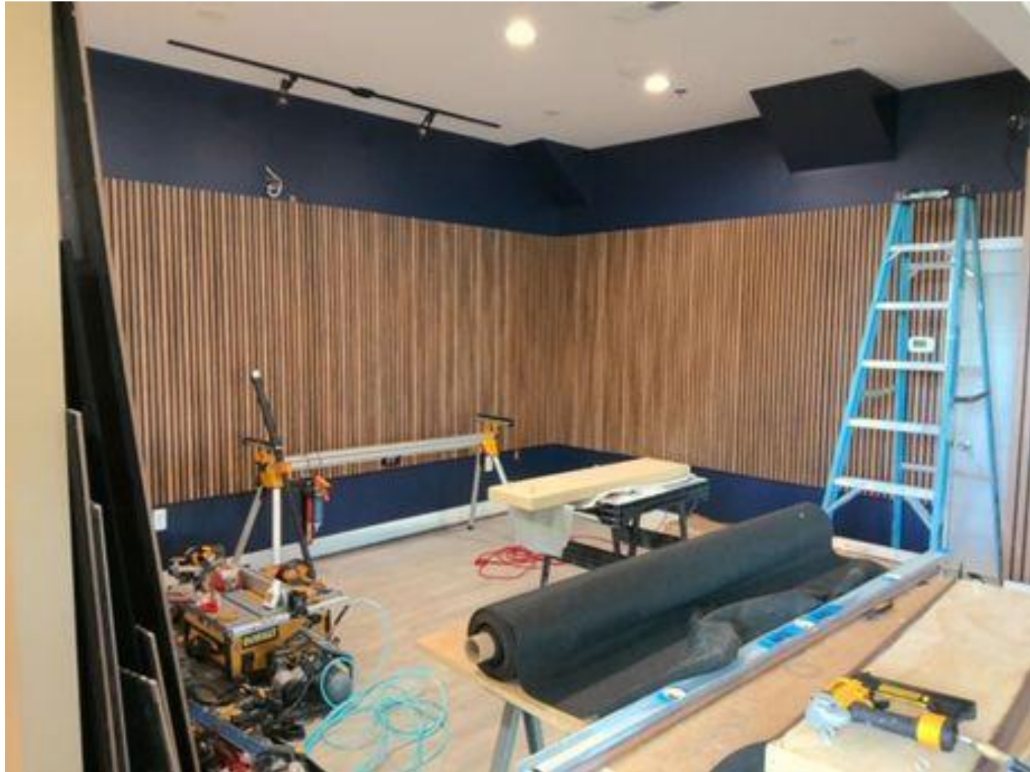
Looking to the left side of the second floor bar area
