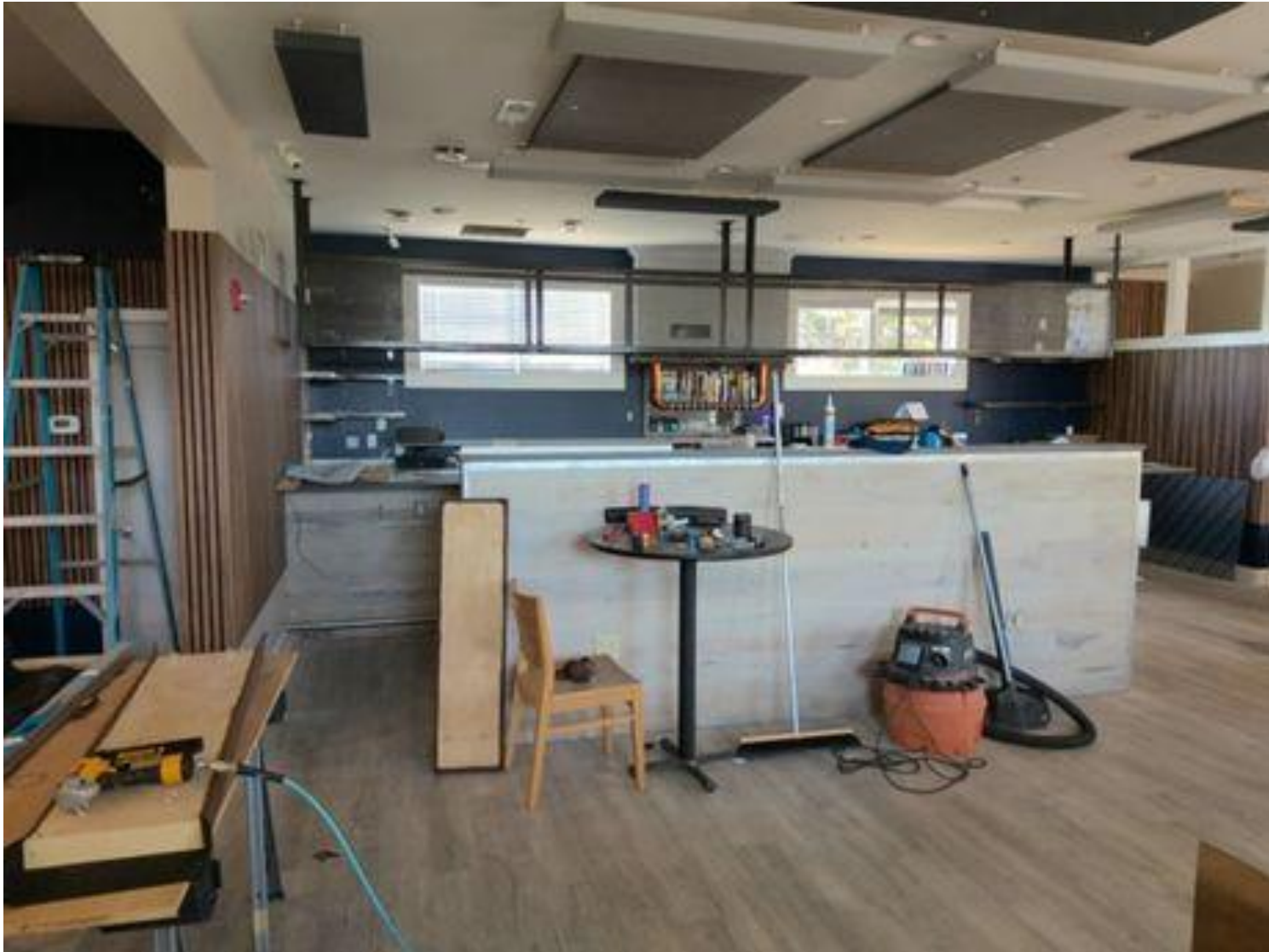
Second floor looking from top of stairway looking towards the bar
