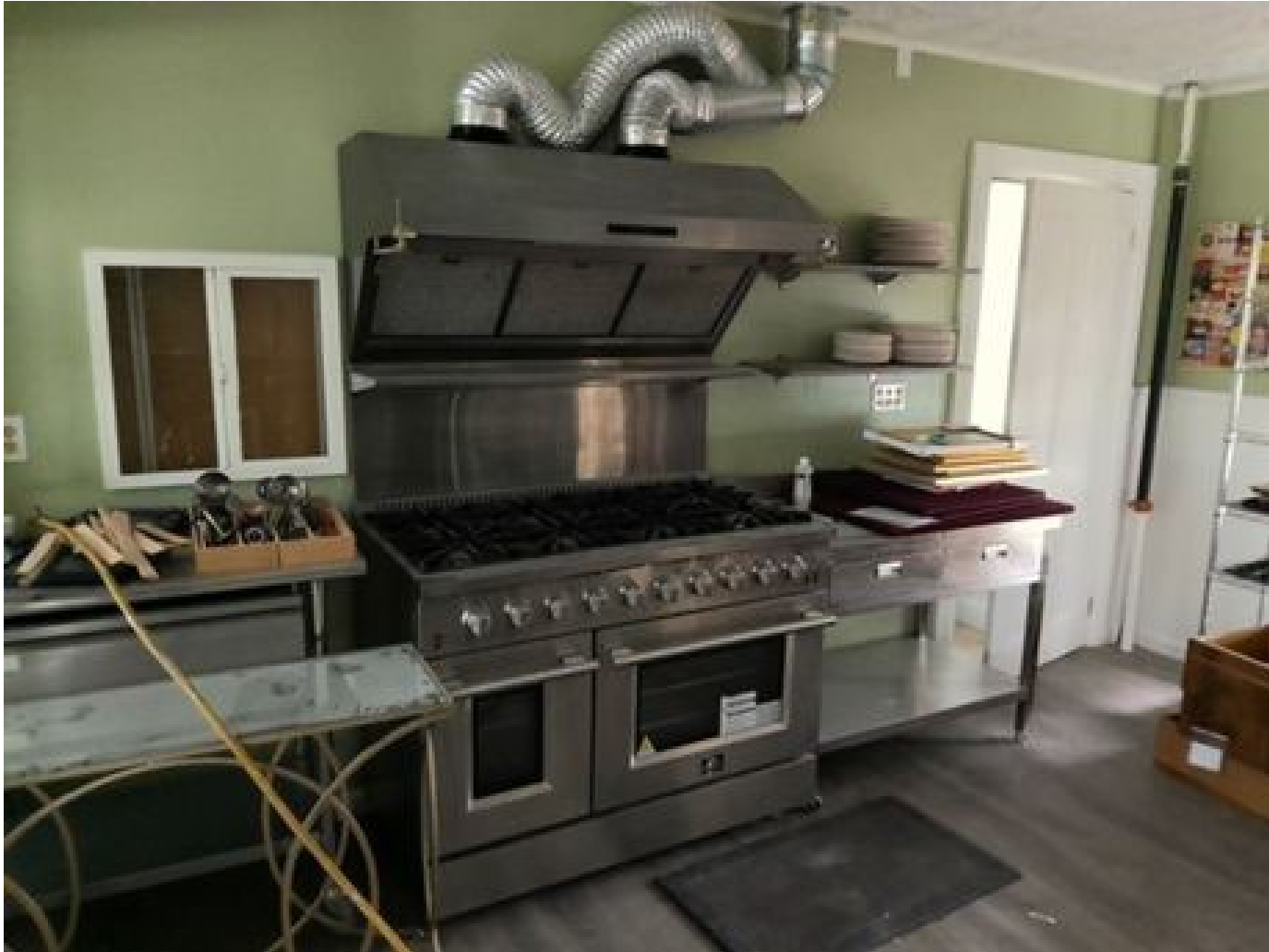
Commercial kitchen area -#1
